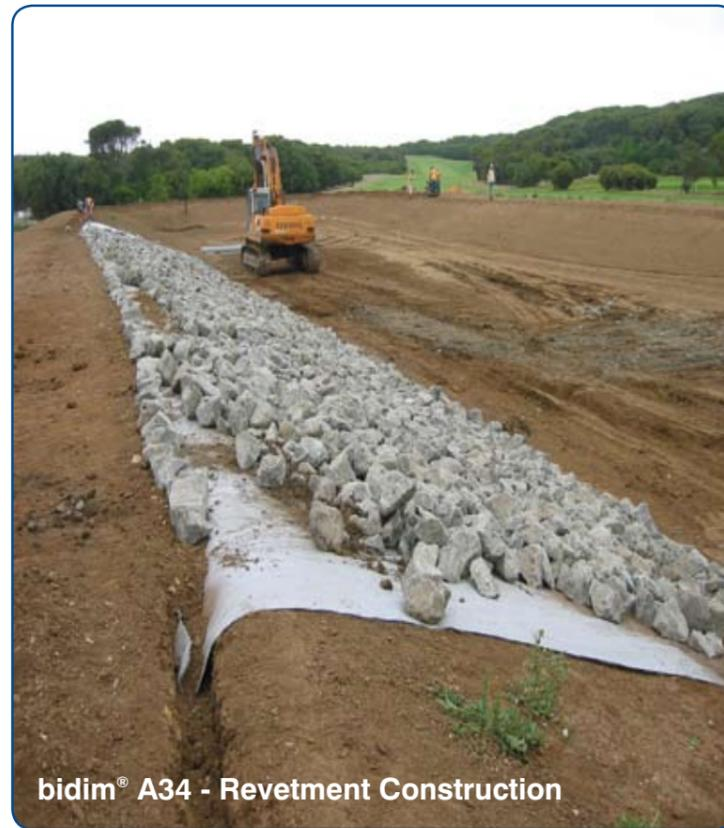
bidim® A34 - Revetment Construction
